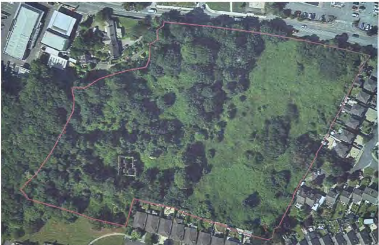
Figure 1.1: Site Location – Fernhill House, Dublin Road, Wicklow Town. The site is located at ITM co-ordinates X 730513 / Y 694546. It is bounded by the Dublin Road, (R750), Glebemount Housing Estate to the south and east, and Trinity Volkswagen / Burkeen Hall to the west.
