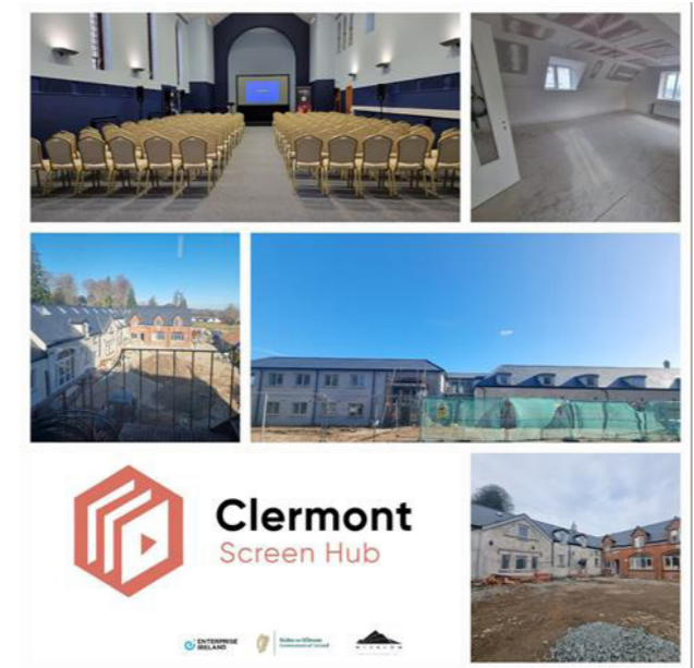
Construction of Clermont Screen Hub
