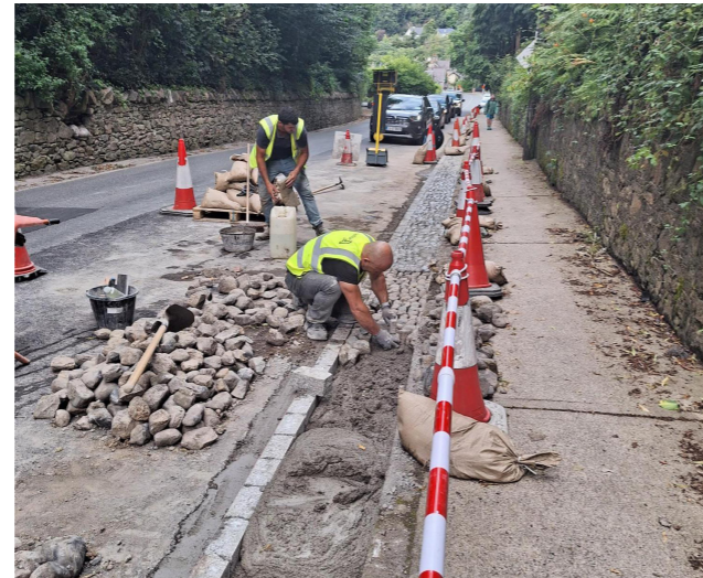
Restoration of cobble channel in Enniskerry
