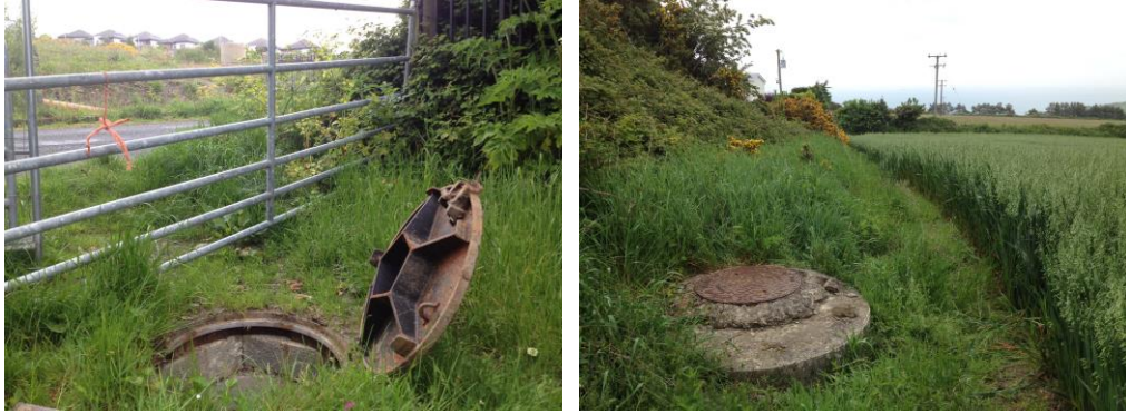
Figs. 4 & 5: Photos of existing foul manholes on the land.
