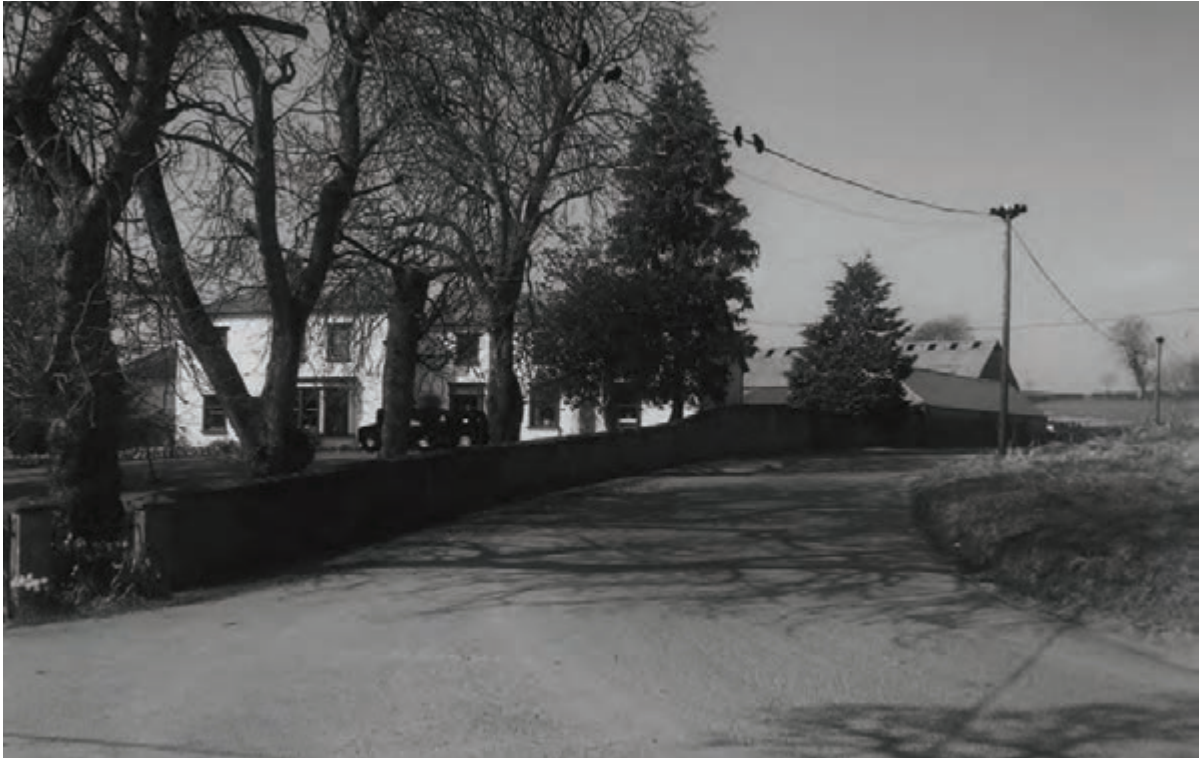
The former Dixon house at Milltown, Dunlavin. Photo taken by the author.
