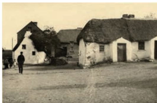
Cottages in the Fishery, Arklow. Photo: Courtesy of Jim Rees
